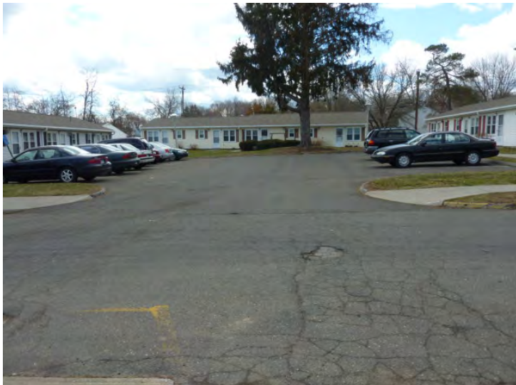
Historic cracking in asphalt paving at sub-base failure.
