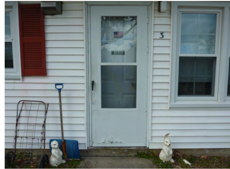
Entry doors and storm doors are well worn and shown to be replaced.
