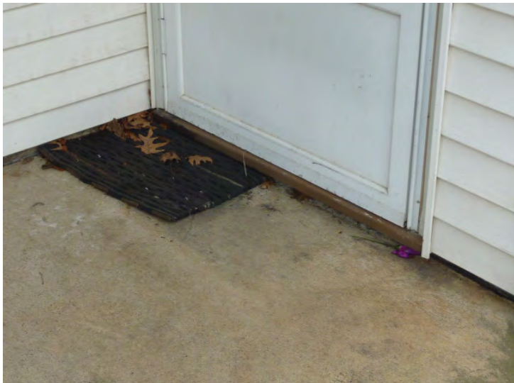
Sill at entry and storm doors has two inch lip and requires a ramp to be part of accessible route.
